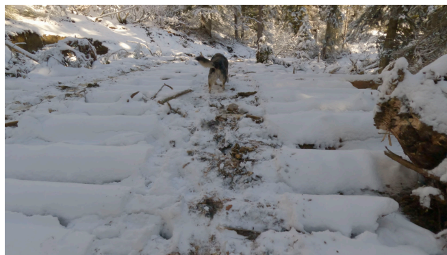
Corduroy road constructed to provide winter access to the central resistivity anomaly and drill hole DD25-TRI-004.
